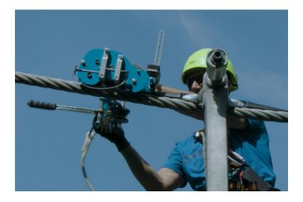
The self-driven carriage is opened by pulling out the lower quick-release pin on the outside. The lower part is opened so far that the carriage can be pushed over the clamp.
