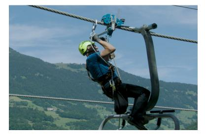
Shortly before reaching an obstacle, the rescuer slowly brakes using the hand brake. The dead man's brake is folded all the way up. The rescuer moves as close as possible to the clamp.
